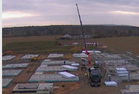
... Transport zur Baustelle
