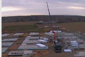
... Transport zur Baustelle
